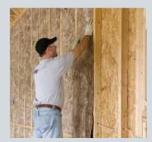
Reduces airborne sound transmission in residential and commercial wall and ceiling applications.
